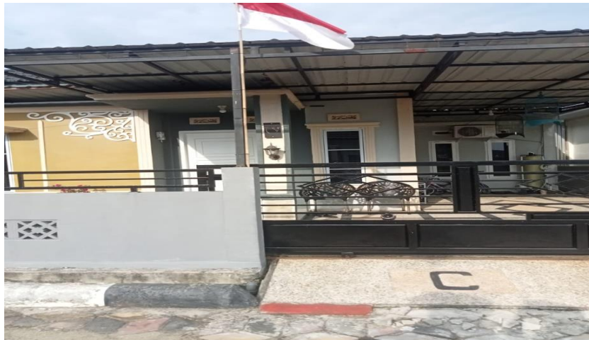
Gambar 4.8 Perumahan Asadel Residence Blok C
