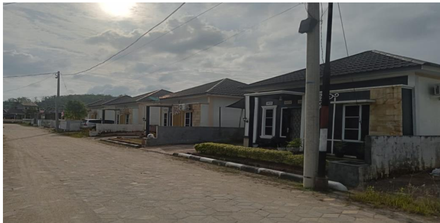
Gambar 4.7 Perumahan Asadel Residence Blok B
