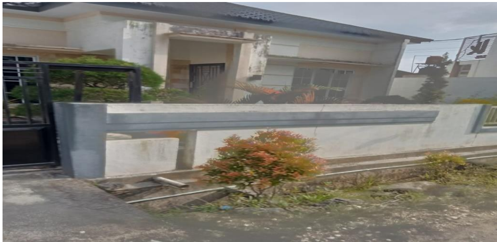
Gambar 4.6 Perumahan Asadel Residence Blok A
